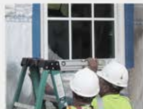
Replacement Windows and Doors, Installations, and Repairs
